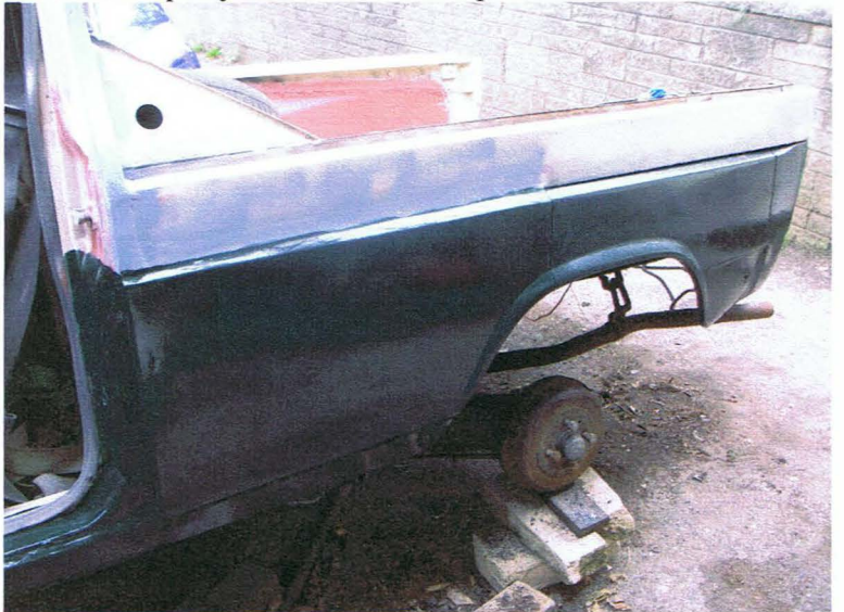
All in place. I've now painted the dark green up to the top of the pickup bed, just leaving the strengthening ribs at the top in beige.
